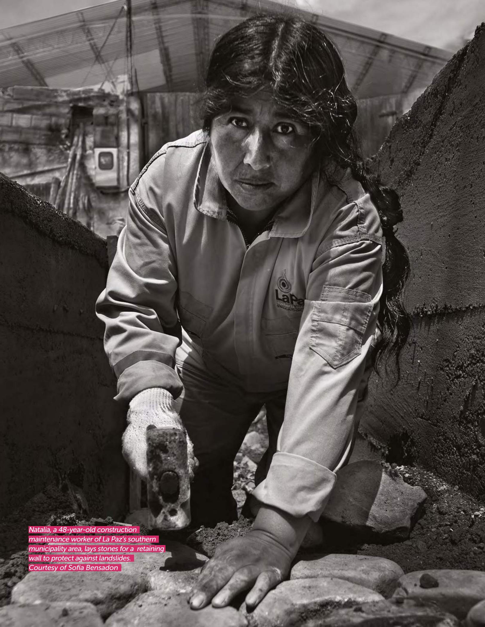
Natalia, a 48-year-old construction maintenance worker of La Paz's southern municipality area, lays stones for a retaining wall to protect against landslides. Courtesy of Sofia Bensadon
